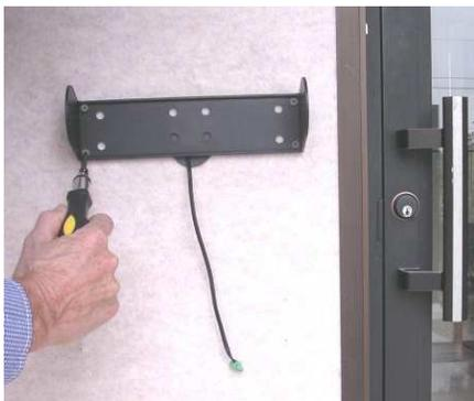
◀ Step 1: Install cable(s) through wall or other convenient routing. Attach the 'U' bracket with appropriate anchors. The bracket can be used as a template to mark anchor spots.
